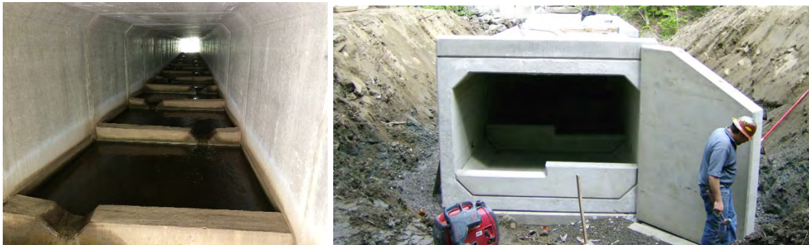
Figure 11: Box Culvert Weir Examples
