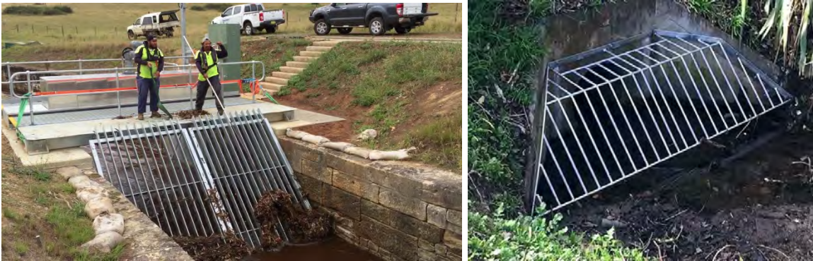
Figure 10: Trash-Rack Examples
